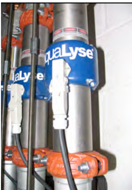
Fig. 4.1.5 - The two connector counterparts are now properly fastened together. To disconnect, simply reverse the order of steps on this page.
