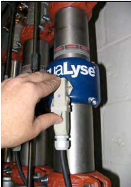
Fig. 4.1.4 - Once both connectors properly inter-connected, the anchor clamp must be used to fasten the cable connector to the ICX chamber cell connector.
