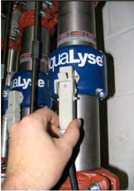
Fig. 4.1.3 - Cable connector can be pushed into the ICX connector once both connectors have been lined up properly. These two components are designed to fit together without great force.
