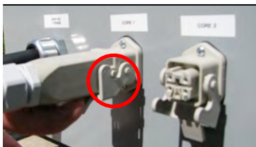
Fig. 4.1.5 - The two connector counterparts are now properly fastened together. To disconnect, simply reverse the order of steps on this page.
