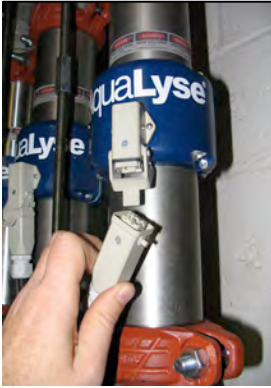
Fig. 4.2.1 - AquaLyse® industrial electrical connectors are clearly identified and correspond to each of required ion chamber cells specific to each model.
