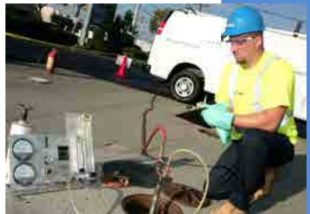
Figure 9.12: Technician performing a tank test
