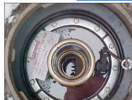
Figure 7.3: View of a flapper valve from a spill bucket
