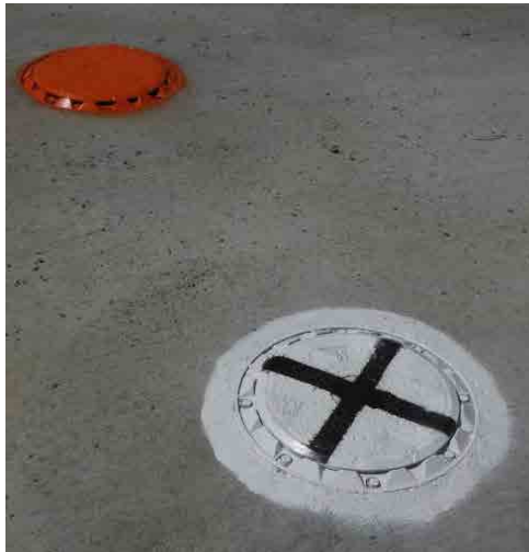
Figure 13.8: Properly colored fill port for unleaded low-grade gasoline (white with black cross) and vapor recovery port (orange circle).
