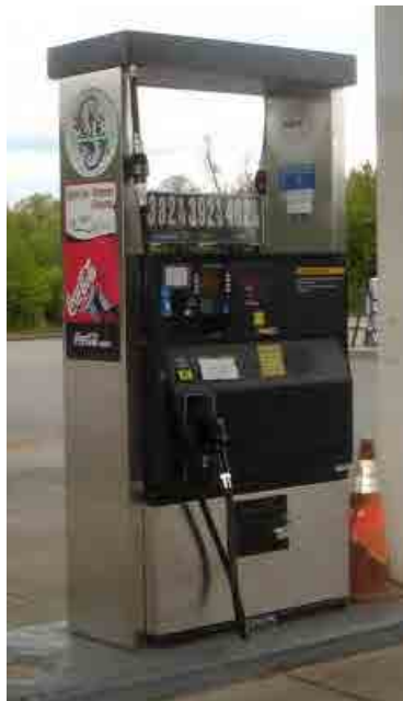
Figure 12.2: Typical retail dispenser providing three different products
