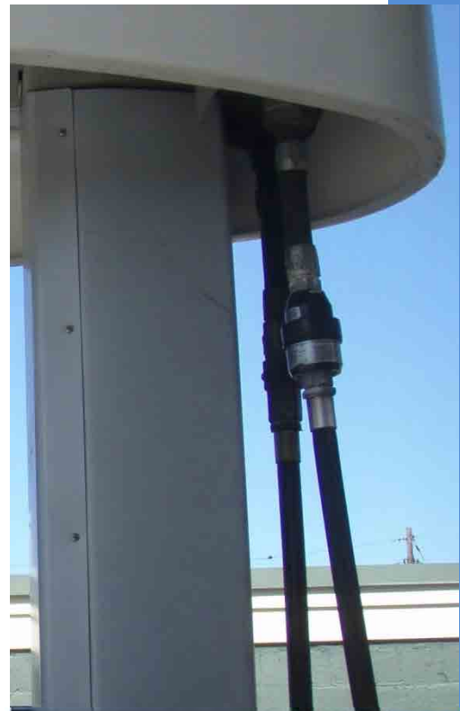
Figure 12.17: Breakaway valve
