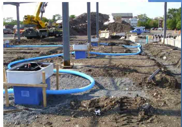
Figure 3.19: Flexible piping during installation
