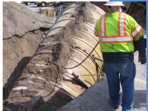
Figure 6.2: Tank Removal
