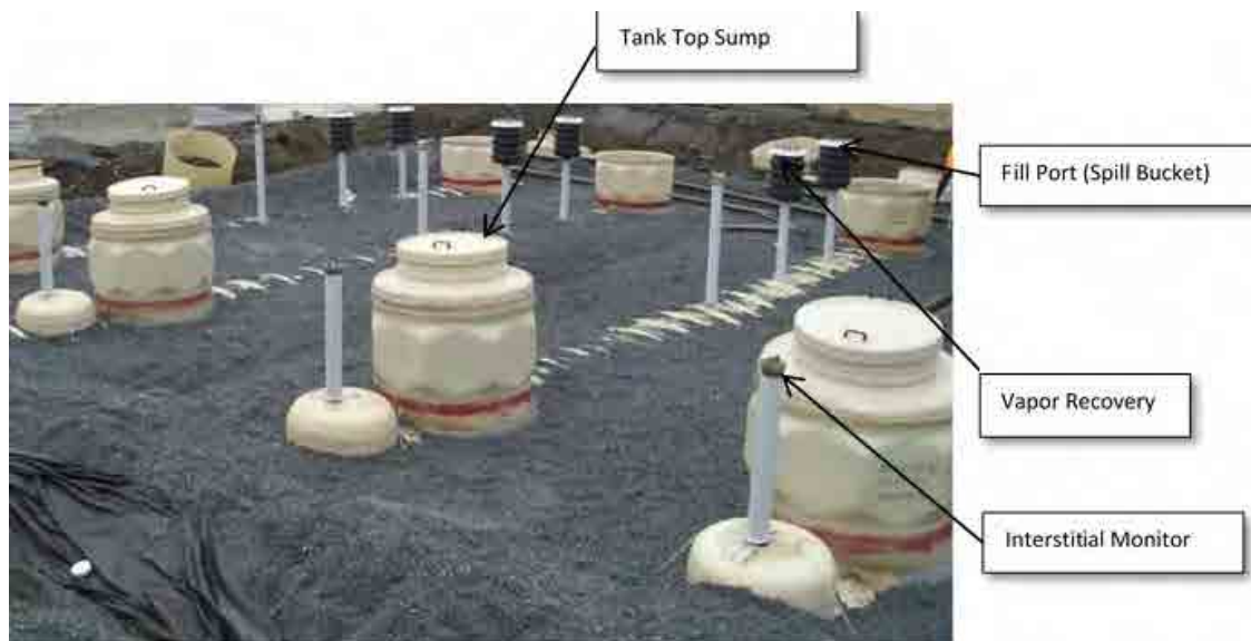
Figure 3.10: Common service station UST layout
