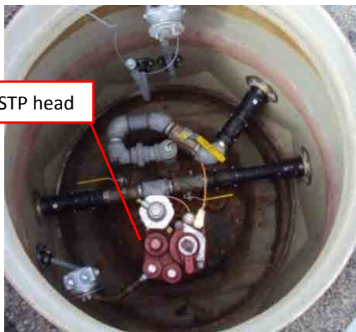
Figure 10.3: Pressurized pumping system
