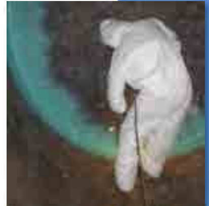
Figure 3.7: Worker spraying a lining on a cathodically protected tank
