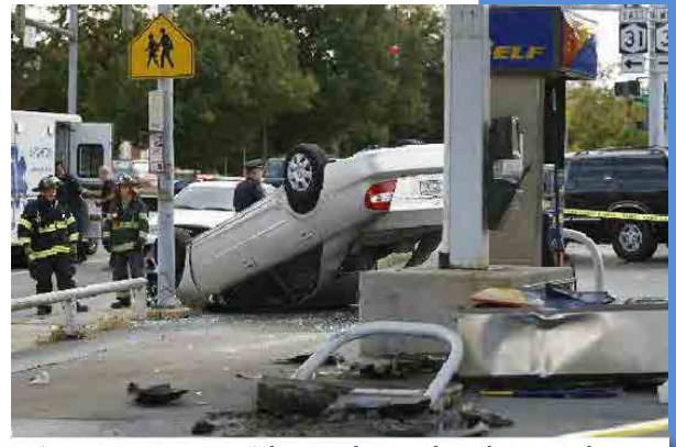
Figure 12.14: Accident where the shear valve properly shut off fuel flow.
