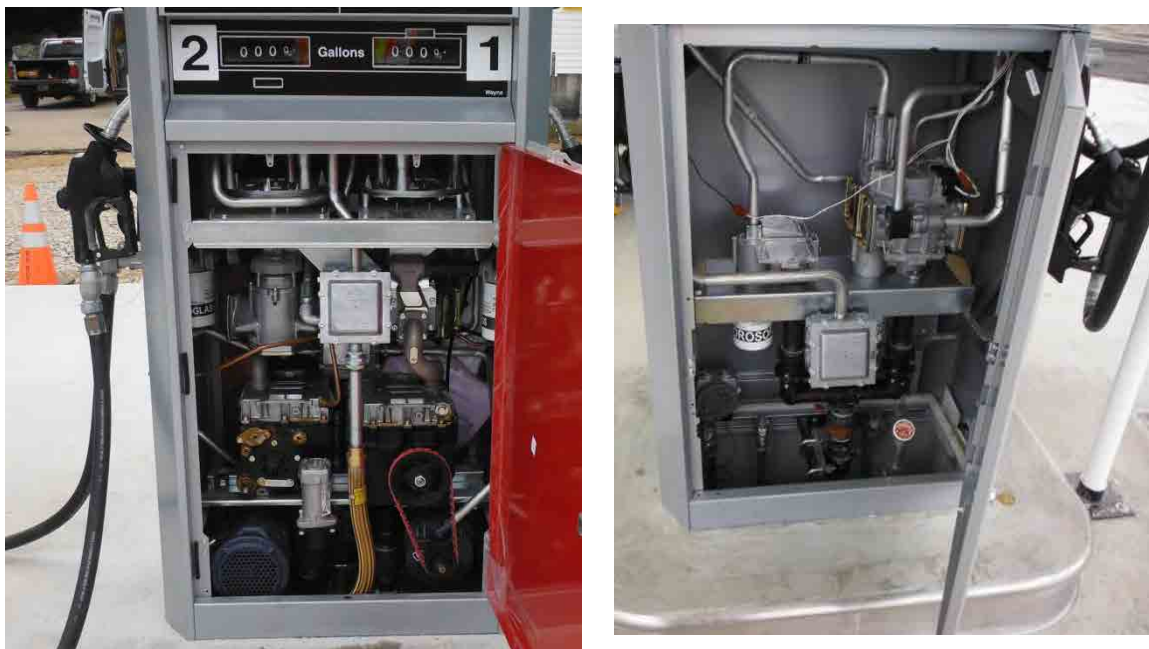
Figure 3.15: Suction system dispenser (left) and pressurized system dispenser (right).
