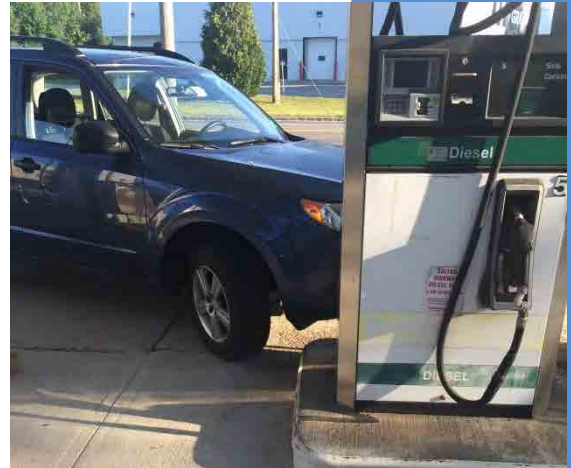
Figure 12.18 Be sure to check your shear valve after an accident such as a vehicle hitting a pump
