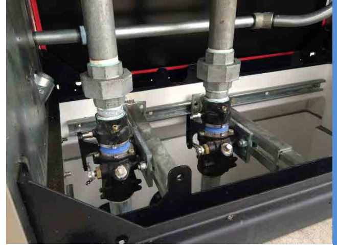
Figure 12.10: Proper shear valve placement
