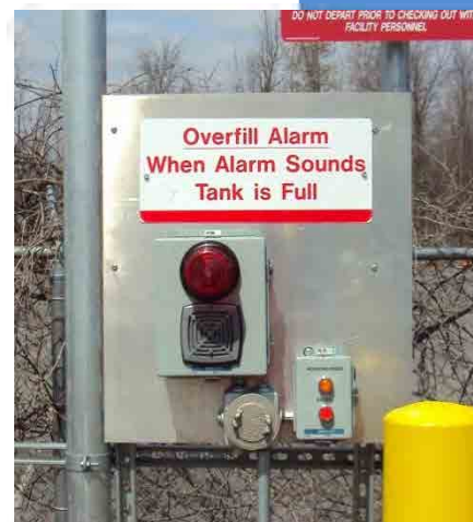
Figure 7.5: Electronic overfill alarm
