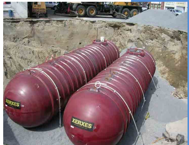
Figure 3.4: Double-walled FRP tank ready for installation
