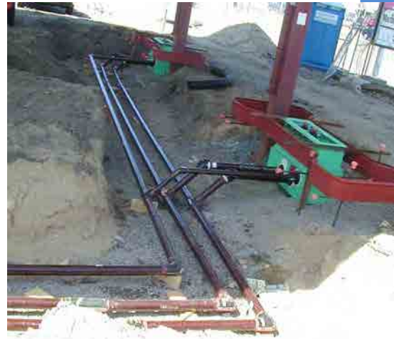
Figure 3.20: FRP piping during installation
