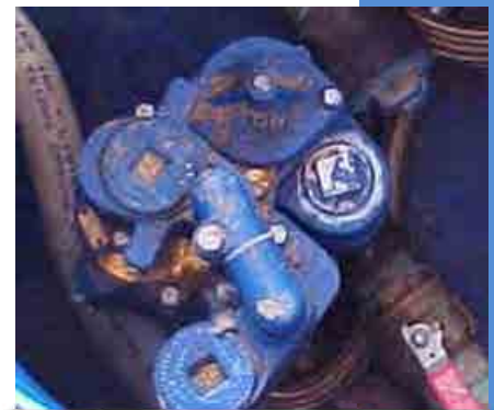
Figure 10.8: Submersible pump with no LLD
