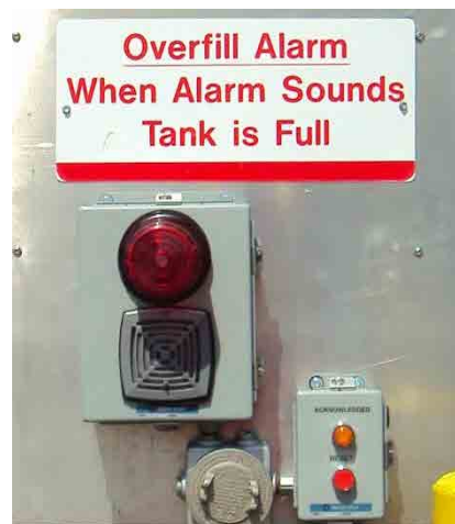
Figure 3.26: Overfill alarm
