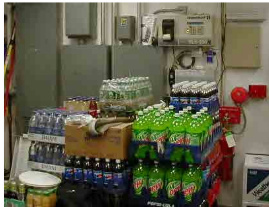
Figure 9.7: ATG console that is not accessible
