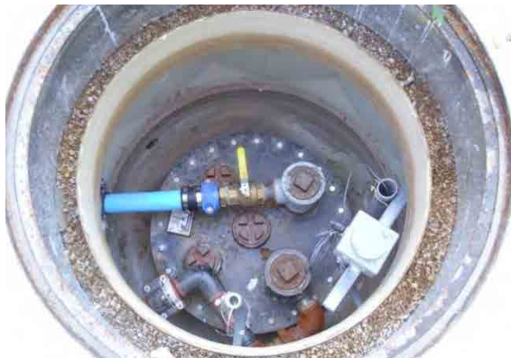
Figure 3.13: Suction piping system
