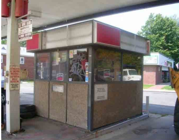
Figure 6.1: Out-of-Service Gas Station
