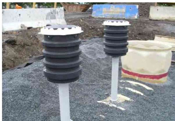
Figure 3.17: Spill bucket
