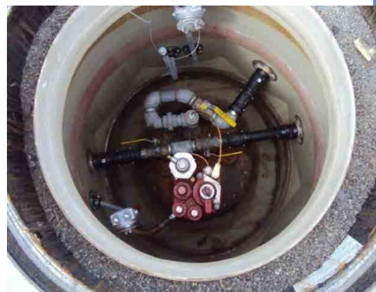
Figure 3.14: Pressurized piping system
