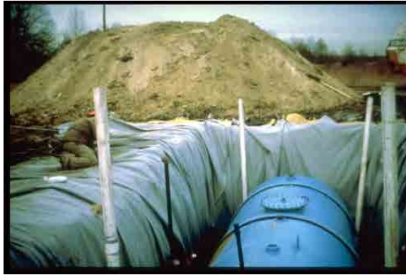
Figure 9.4: Tanks being installed with a secondary barrier
