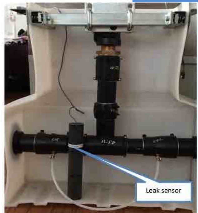
Figure 10.13: Cut-away view of a UDC with a leak sensor and plastic tubing connected to Schrader valves. Note the correct (vertical) orientation of the sensor.
