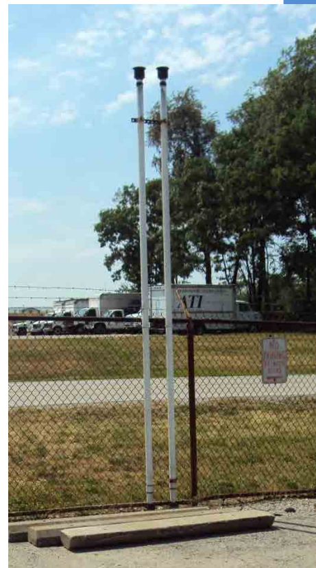
Figure 3.21: Vent stack arrangement
