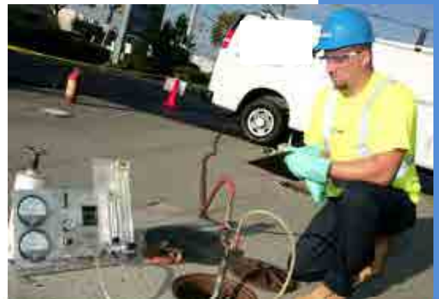
Figure 14.7: Technician performing a tank test
