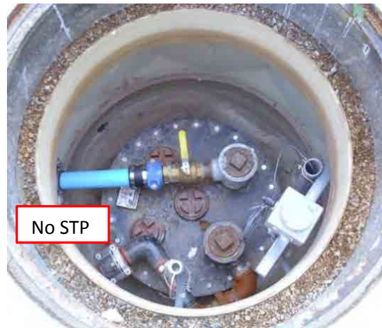
Figure 10.4: Suction pump system
